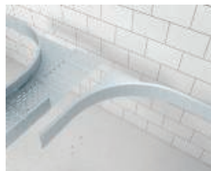
T-hargnemiskoha loomine nurgadetaili abil Teise nurgadetaili WEAS 110 paigaldamine.
